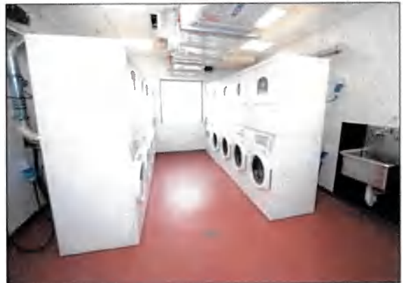
HDF Laundry Room
